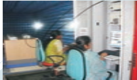
IM3 testing using Passive Inter-modulation Analyzer
